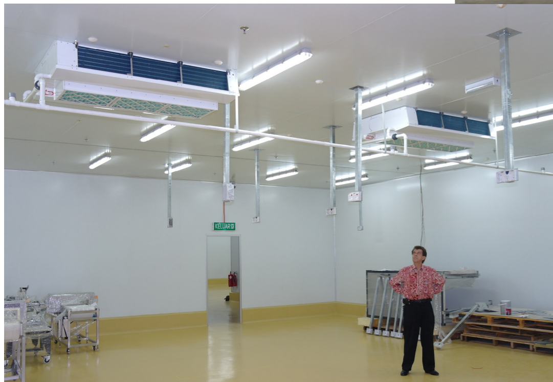
Dual air discharge units. 16 °C Processing room
